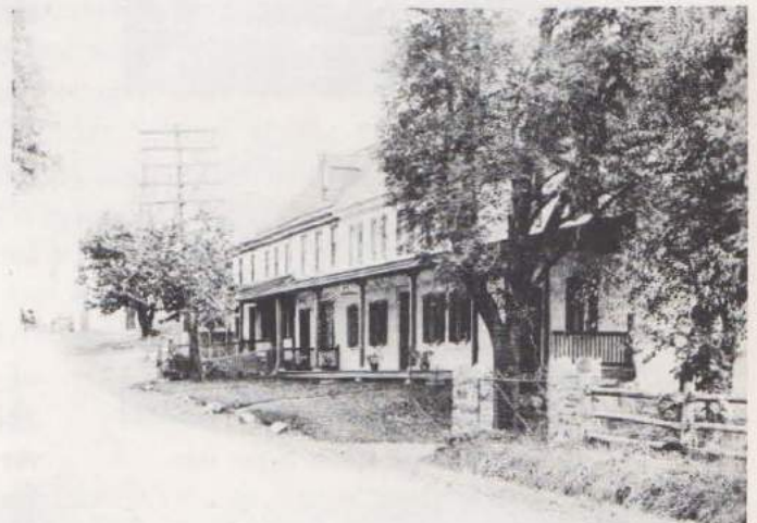
Then: Lancaster Avenue 1910, looking east into Radnor Township. Sarah Siter's house is the nearer of the buildings.
