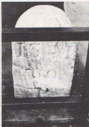
The 13th milestone on the Philadelphia and Lancaster Turnpike.
