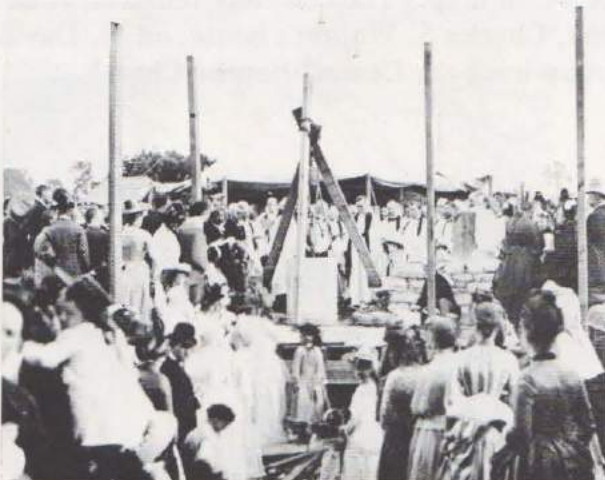
Laying the cornerstone of St. Mary's Church June 27, 1889. The Rectory, to the east, became the Radnor Township Building in 1928. Wilson Brothers and Company designed the Church. (See 70 on map.)
