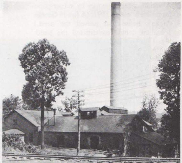
The Wayne Steam Heat Plant in 1908. Built about 1895, it operated until 1948. (See 47 on map.) A similar plant, built by Wendell and Smith in Overbrook, lasted until the 1970's.
