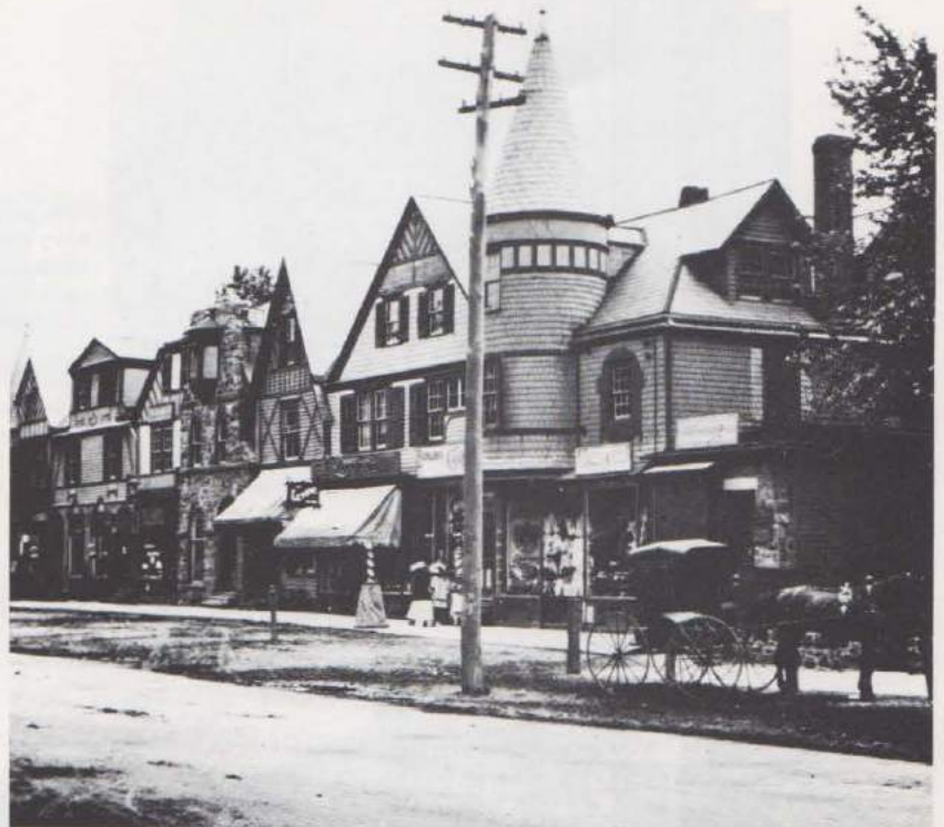
The Wayne business block in 1890, when new. Note the barber pole by the second store. The block stands, minus the towers. (See 52 on map.)
