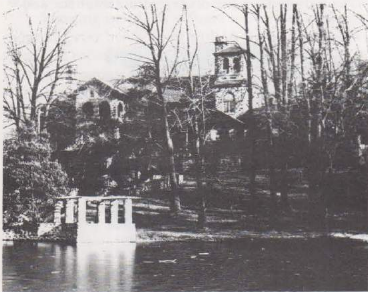
Waltharthon, designed by David Knickerbacker Boyd, built in 1913, pictured in 1975. Now the property of Eastern College. (See 64 on map.) my home to use part of their dormitory on Eagle Road.
