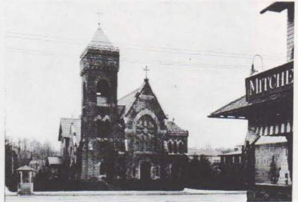
St. Katharine of Siena Church, dedicated August 30, 1896, as it appeared in 1934. It was razed in 1965 in favor of a new building. (See 73 on map.)
