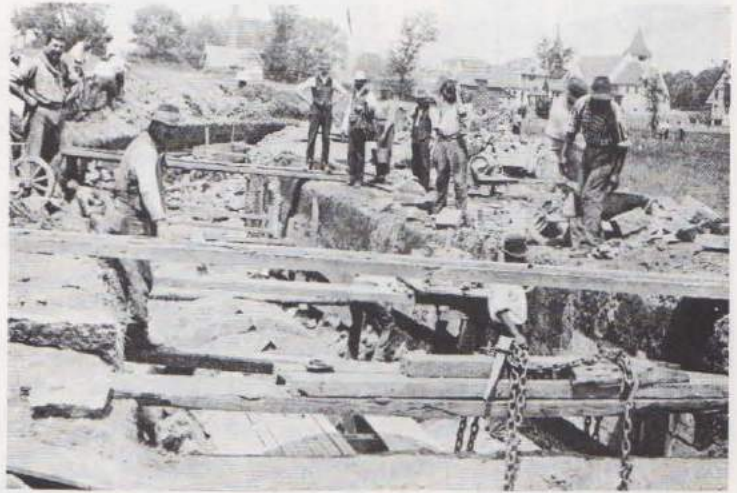
Laying drains on Aberdeen Avenue in 1890. (See 44 on map.)
