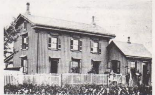
Station (all) and station master's house about 1875. (See 18 on map.) Last used as a dormitory for Wayne Hotel waiters, the house was razed for parking space.
