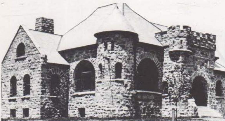
Wayne Title and Trust Company when new in 1890. The present building replaced the old in 1930. The Law Offices of Greenwell, Porter, Smaltz and Royal have occupied the second floor for more than 30 years. (See 59 on map.)
