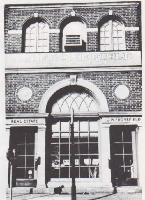
105 West Lancaster Avenue, built 1928, picture in 1975. (See 50 on map.)
