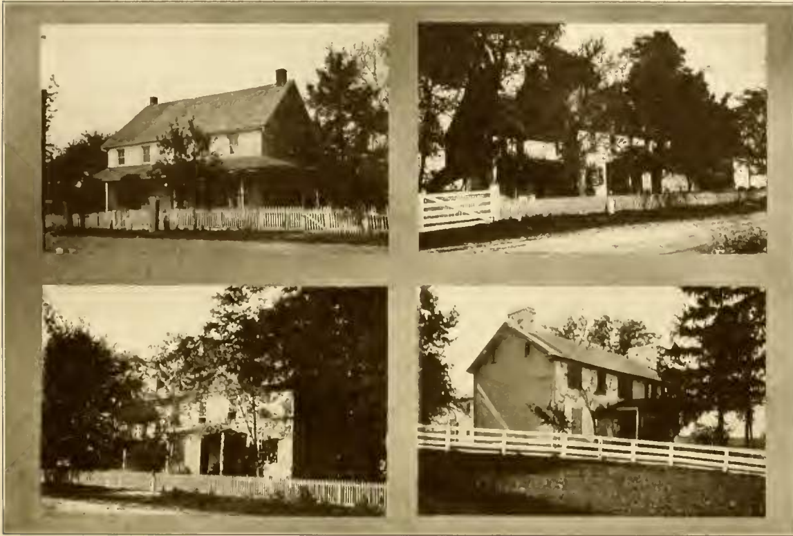
THE LANCASTER TURNPIKE AT 43 d MILESTONE—"OLD MOSCOW."
